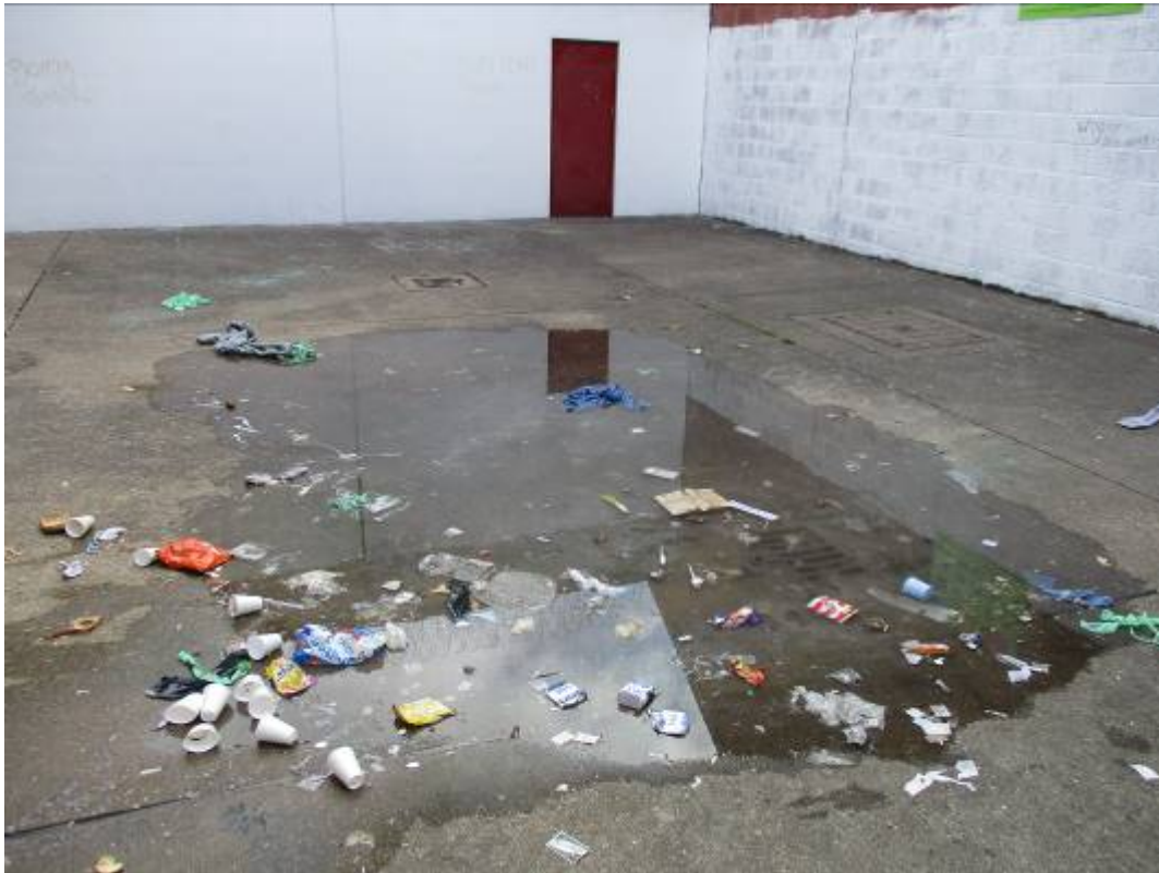
Segregation exercise yard
