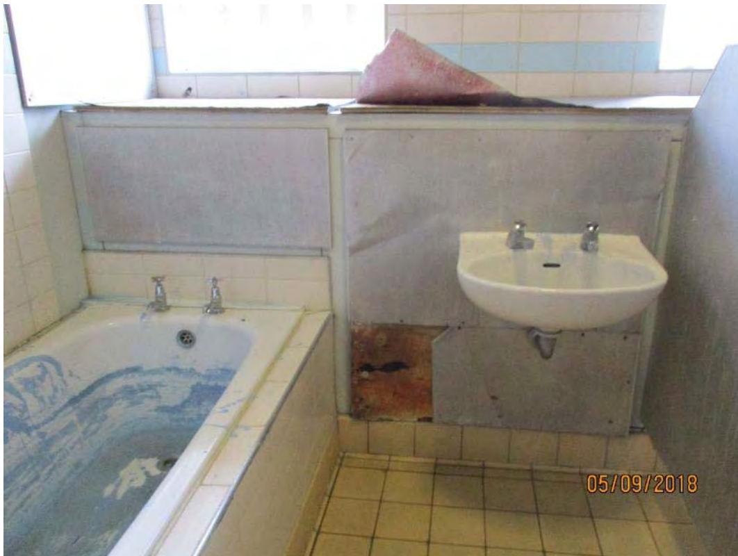
Photograph 2. D wing shower room
