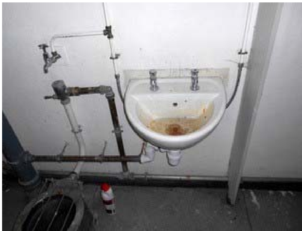
Communal toilet and shower area on C wing
