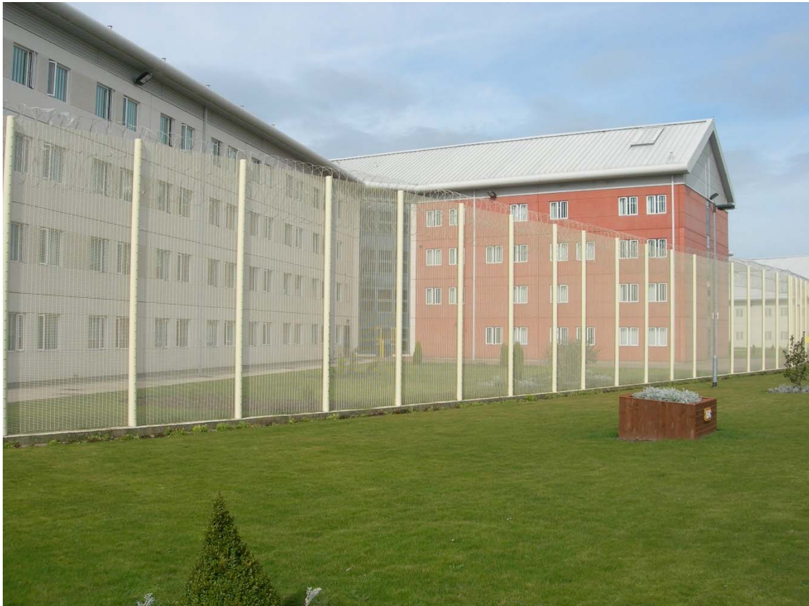
The impressive and well-maintained external areas.
